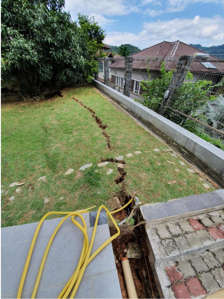
Tension crack
